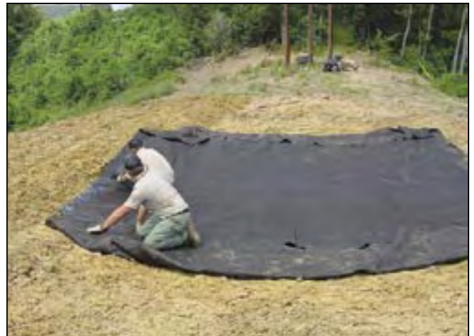
A liner is placed in the depression.
