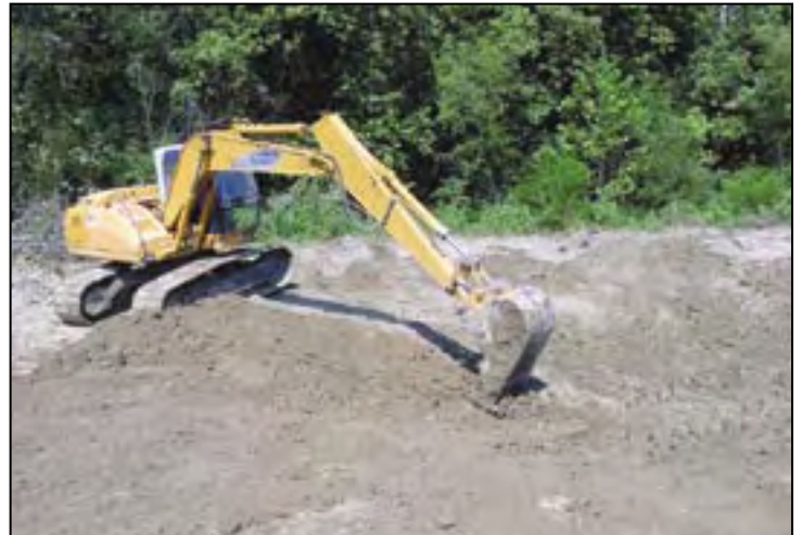
This track-hoe is being used to make an ephemeral wetland. These machines are also used to drain natural wetlands.
