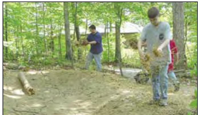
They seeded and mulched the exposed soil.
