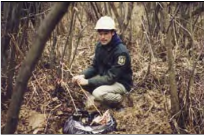
AN/FO is placed in a shallow hole.
