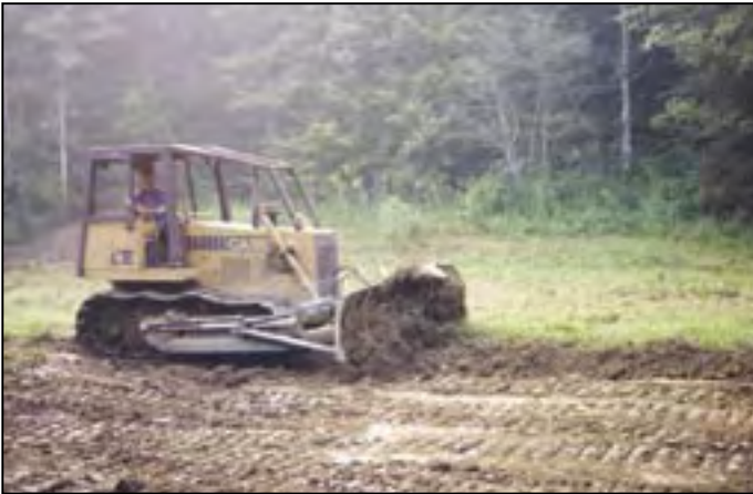
Remove and save topsoil.
