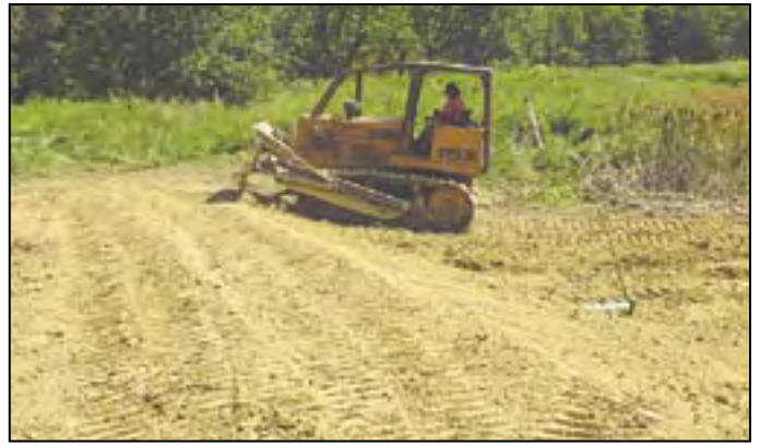
Pack the dam in layers.
