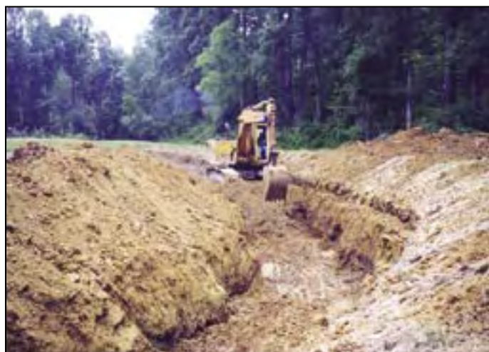
As the trench is being dug, silt loam is placed inside the wetland; gravel outside the wetland.
