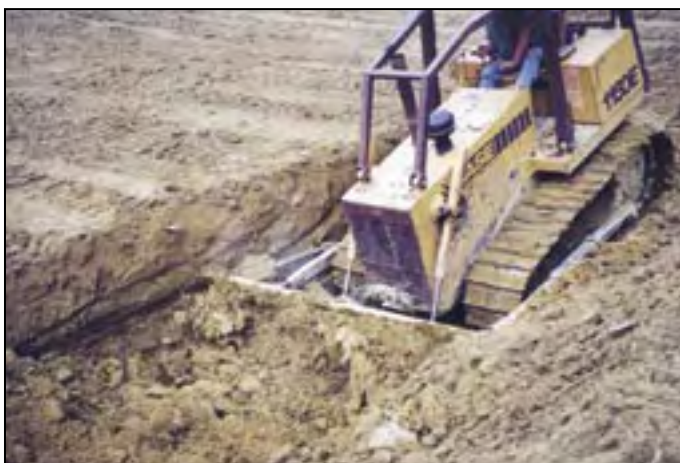
Dozer moves and packs soil in the core.
