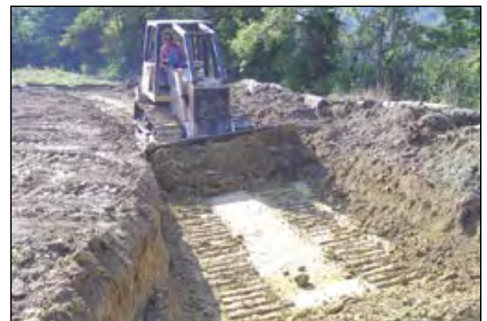
Core is located under the entire dam.
