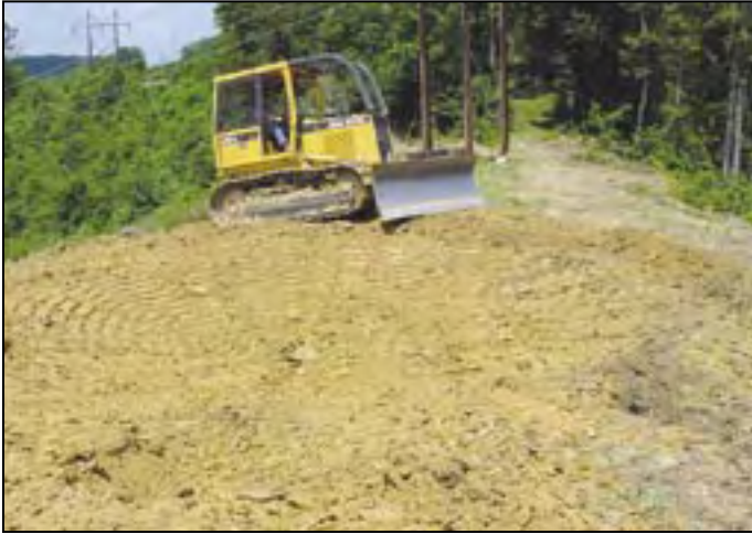
A dozer makes a shallow depression in the soil.
