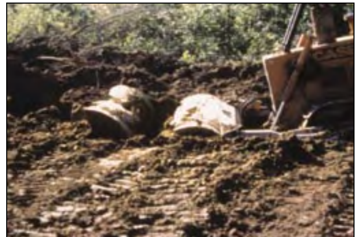
Dozer moves soil in the core to eliminate holes.
