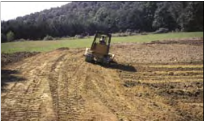
Make gradual slopes on the dam.
