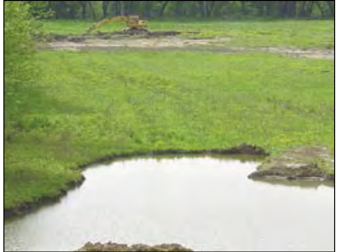
This vernal pond was built with a track-hoe on a site with a high water table.
