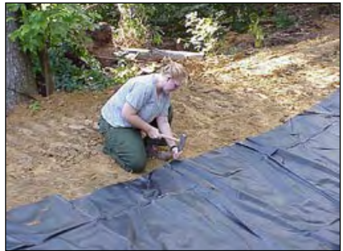
The liner is secured with stakes.
