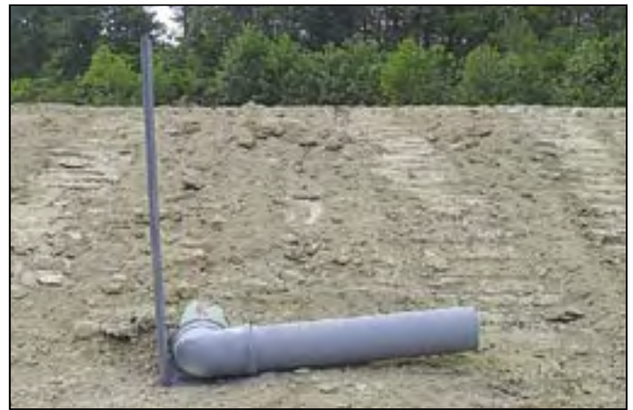
The same pipe can be moved parallel to the ground to drain the wetland.
