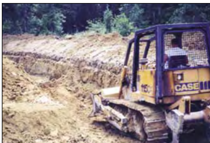
Dozer fills the core trench with silt loam.
