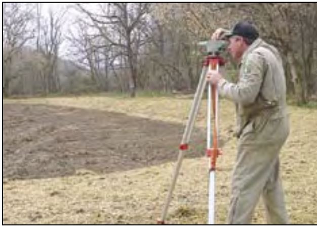
Using a level to measure slope on a vernal pond construction site.
