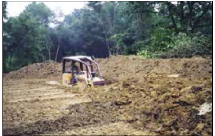
Make a core under the dam location.
