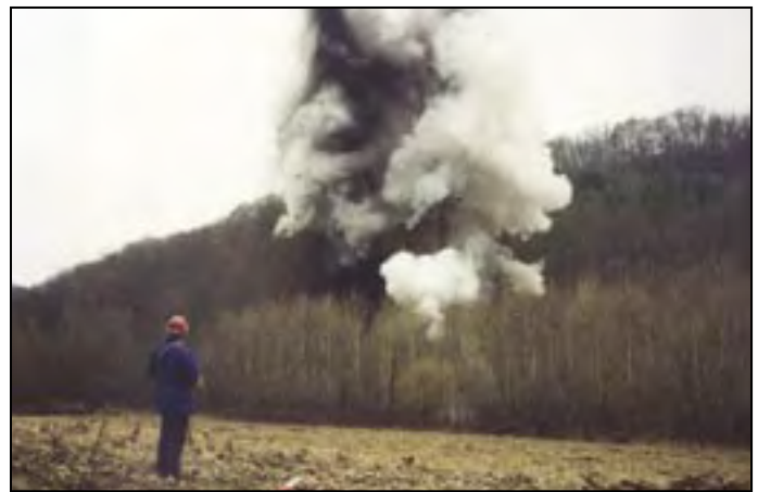
A licensed blaster detonated the AN/FO.
