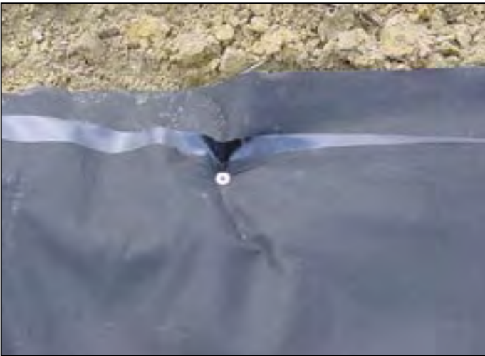
The liner is protected on both sides by geotextile fabric.
