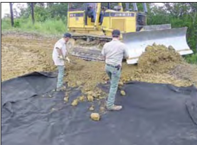
A dozer is used to cover the liner with soil.
